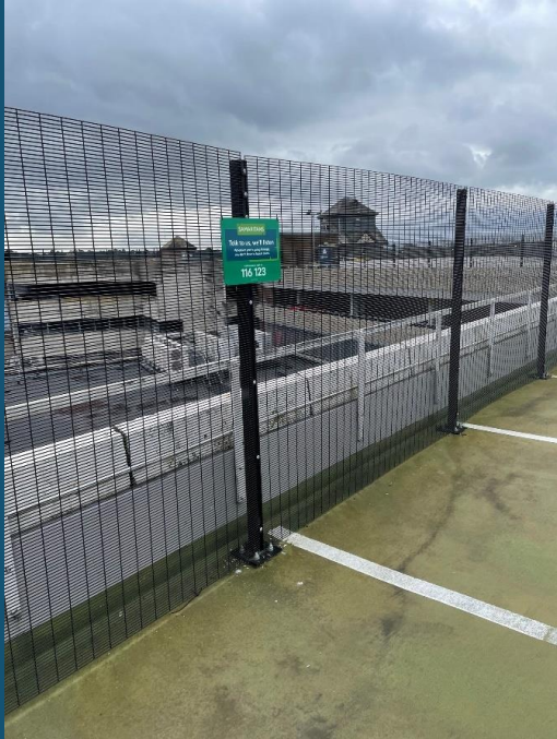
Photo- Anti-trespass fencing with Samaritans signage
