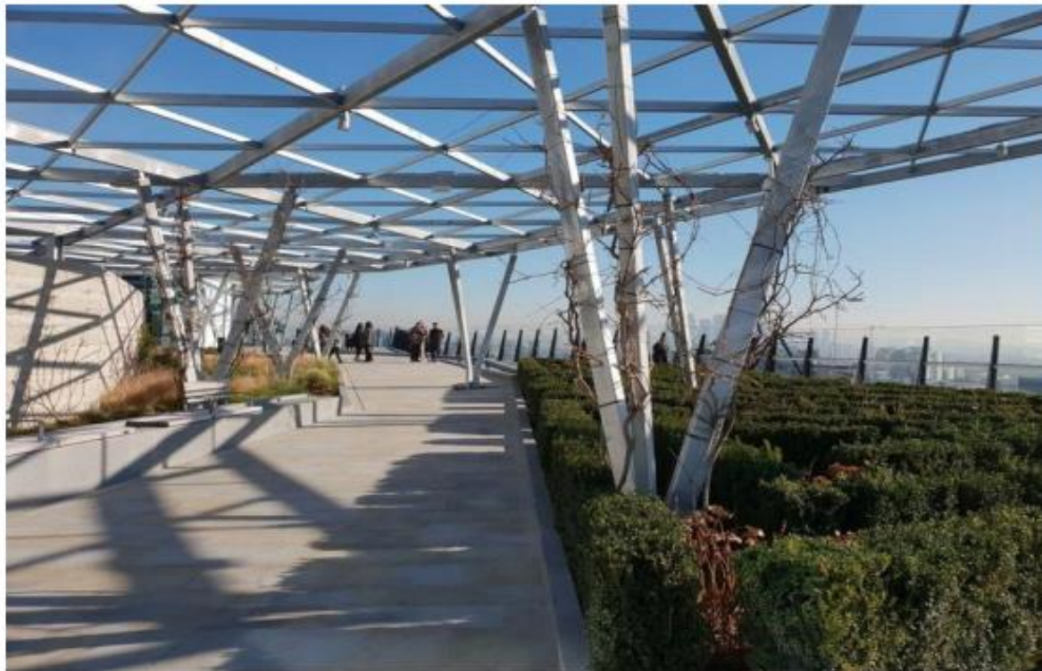
Planting on roof terrace at 120 Fenchurch Street
